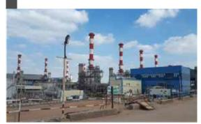
**Plant Description:** Two combined cycle modules, Consists of 8 units GE Frame 9E gas turbines (Each of 125 MW), 8 HRSGs and 2 steam turbine units.
