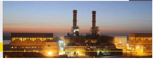
Plant Description: Kurimat power project consists of two modules each module includes two 250 MW combustion turbine generators (CTGs). Each one feeds exhaust gases to its respective heat recovery steam generator (HRSG). Steam from two HRSGs feeds one 250 MW, reheat, condensing steam turbine generator (STG).
