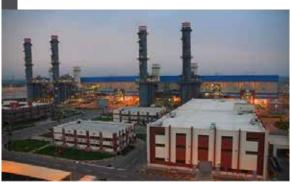
Plant Description: Nubaria power project consists of three modules 750 MW comprised of two 250 MW combustion turbine generators (CTGs). Each one feeds exhaust gases to its respective heat recovery steam generator (HRSG) with no supplementary firing. Steam from the two HRSGs is fed to one 250 MW.
