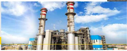
Plant Description: Banha power project includes a power block that consists of two 250 MW Combustion Turbine Generators (CTGs). Each one feeds exhaust gases to its respective unfired Heat Recovery Steam Generator (HRSG). Steam from the two HRSGs feeds one 250 MW, single reheat, condensing Steam Turbine Generator (STG).
