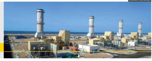
**Plant Description:** West Damietta power project is a simple cycle power generation project located within the vicinity of the existing West Damietta power station. It consists of 4 outdoor gas turbines with a total capacity of 500 MW.
