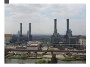
Plant Description: Cairo North power project includes a power block that consists of two 250 MW combustion turbine generators (CTGs). Each one feeds exhaust gases to its respective heat recovery steam generator (HRSG). Steam from the two HRSGs feeds one 250 MW (nominal), reheat, condensing steam turbine generator (STG).
